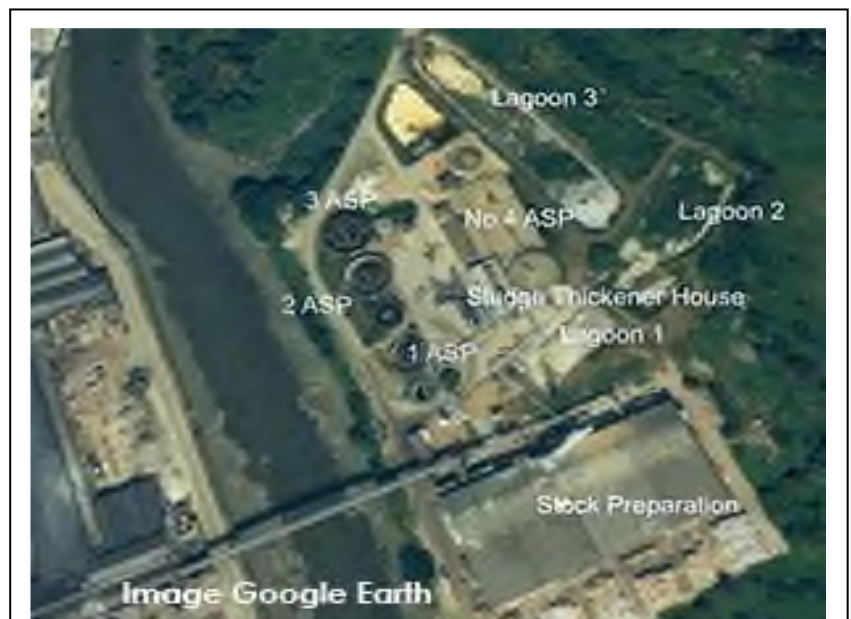
Figure 5 Effluent Plant - Island Site
